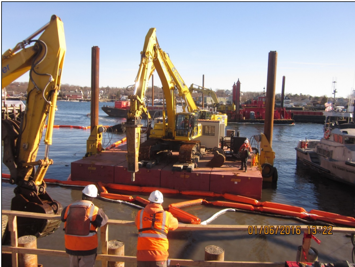
Figure 8: Excavator with a Jackhammer.
